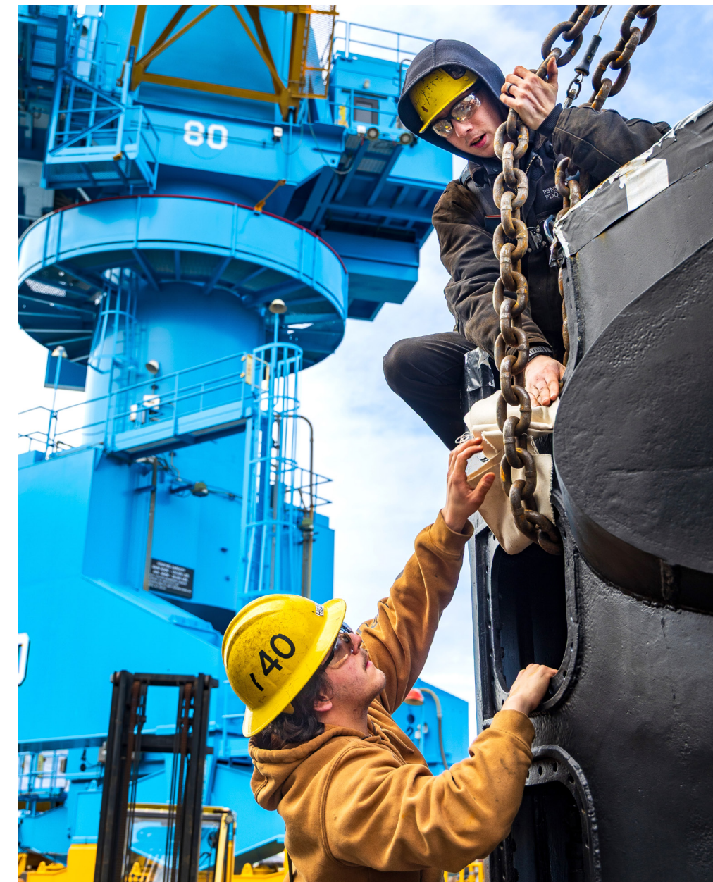
ABOVE: Alexander Hackett, right, and Ethaniel Hiller, both riggers, Code 740, Riggers, work together to hook up rigging gear in preparation for Ex-Norfolk's sail to be lifted onto a flatbed trailer, Feb. 24.
