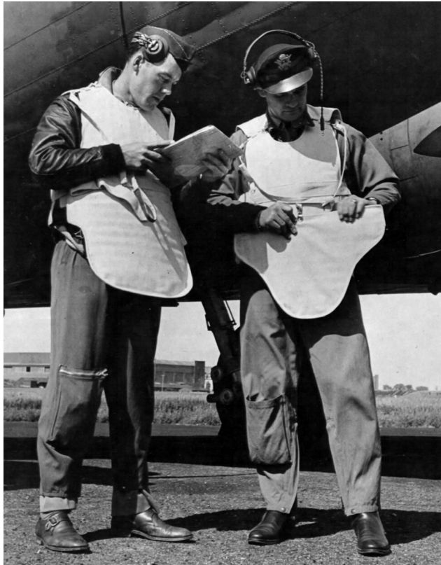
Above and Top Right: Aircrew armor. Aprons could be detached and the vest worn alone for seated airmen.
