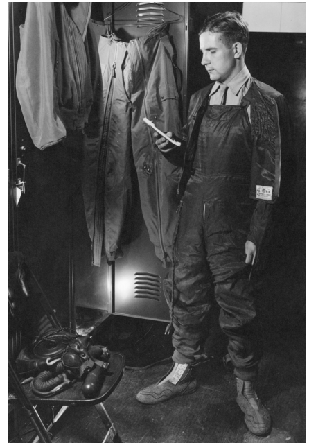
Above: Views of the late-war, two-piece Type F-3 Electric Suit
