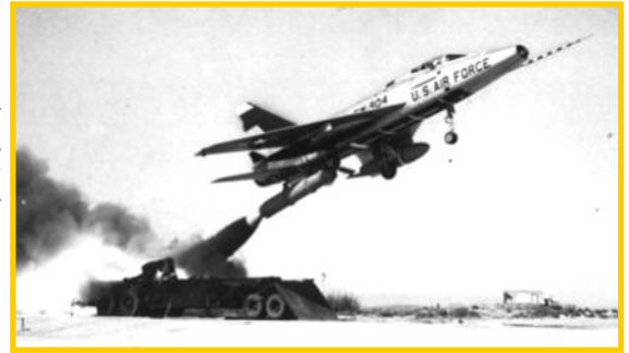
A North American Aviation F-100 performs a zero-length launch during early testing.
