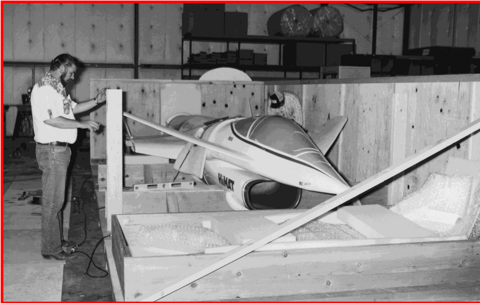
The second mockup, constructed from wood and fiberglass, gave an accurate representation of the actual vehicle. Crated at Rockwell and shipped to ADFRF, the mockup could be shown to visiting dignitaries. This mockup is currently stored at the Air Force Flight Test Center Museum at Edwards AFB, CA, awaiting restoration.
