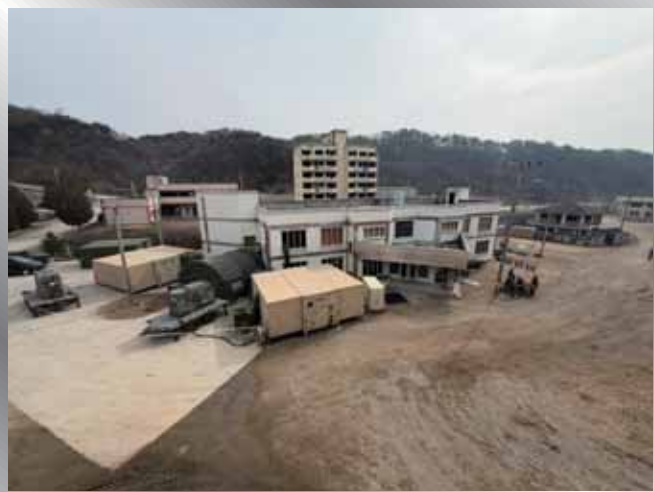
502D Field Hospital established in a building of opportunity
