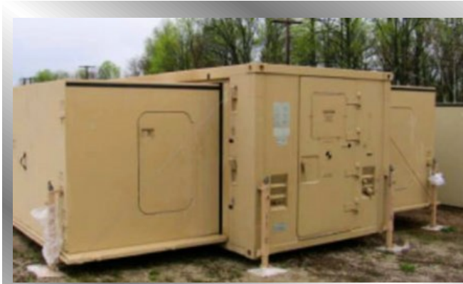
Shelter, Tactical, Expandable, Two Side (ISO Container) regularly used in the field environment that will soon be attached to the BDAACH facility.
