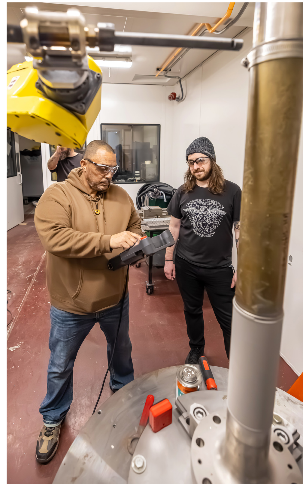
ABOVE: Alan Tomlinson, right, additive manufacturing supervisor, Shop 31, Inside Machinist, works with shipyard contractor Robin Mesa April 14, during a recent repair procedure inside the cold spray booth in Building 431 at PSNS & IMF. (U.S. Navy photos by Jeb Fach)
