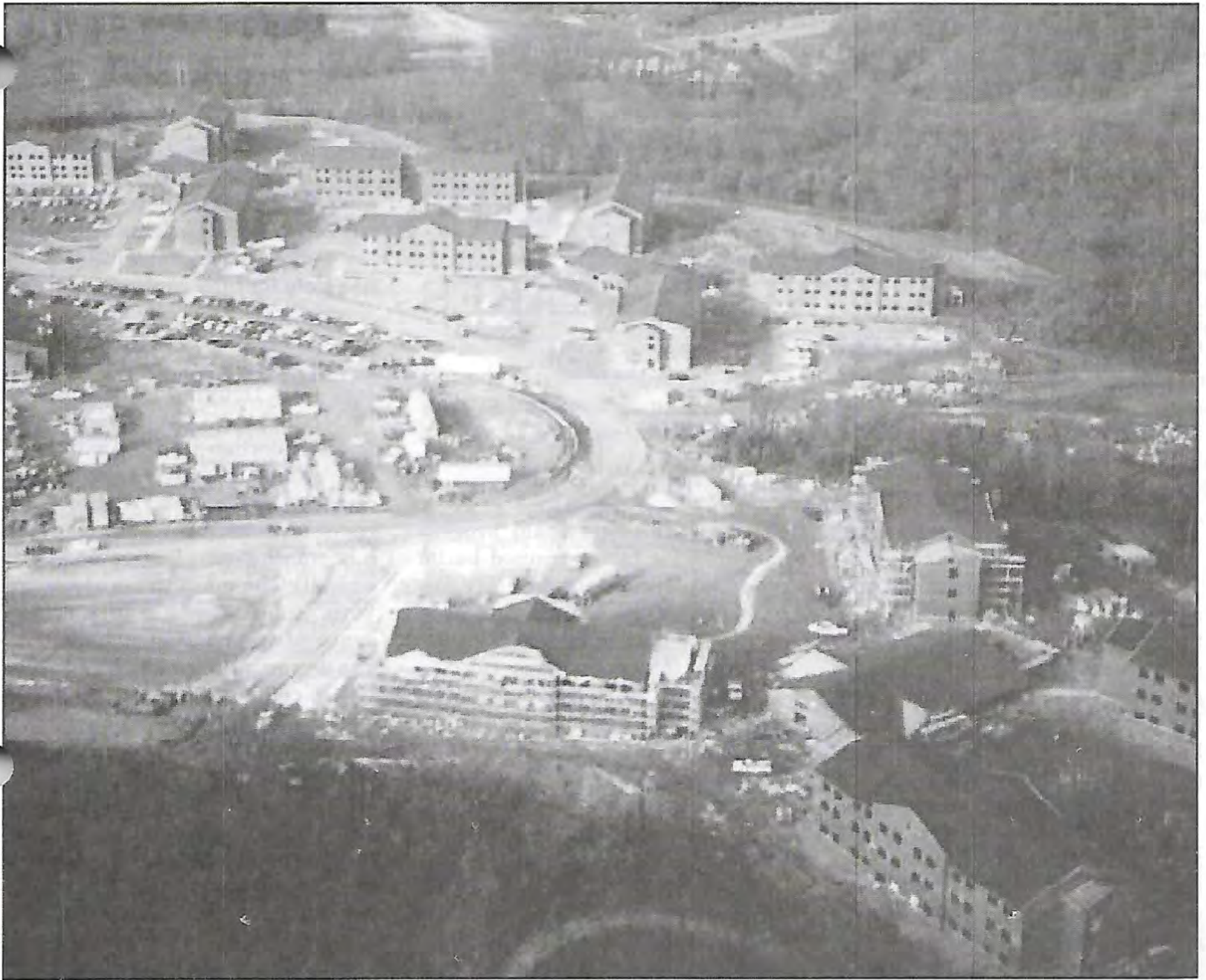
Figure 8. Construction Site of the Unaccompanied Enlisted Personnel Housing (UEPH)
