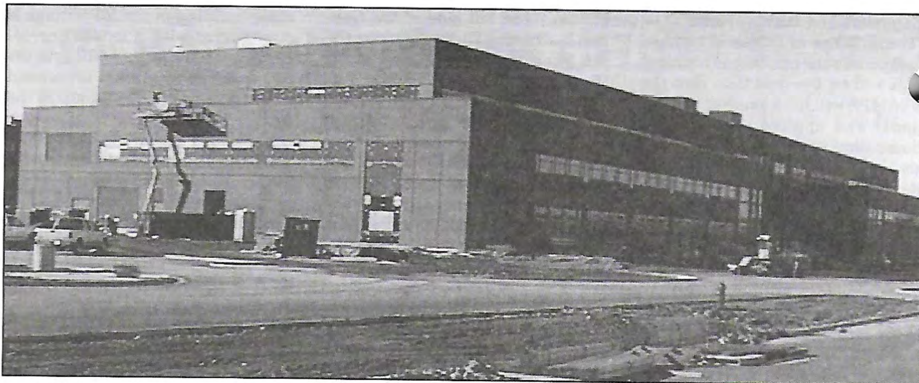
Figure 2. General Instruction facility
