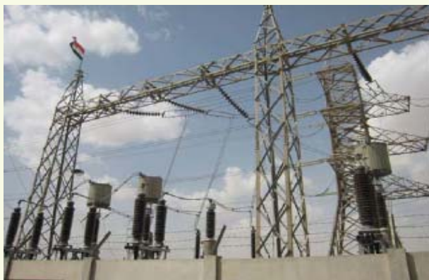
Transformers at the 132 kv substation at the Port of Umm Qsar.
