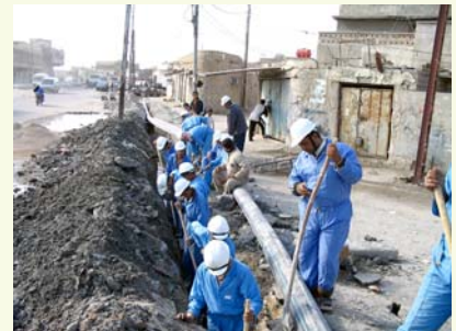
Iraqi civilians have installed 200 kilometers of water pipes made of high-density polyethylene.
