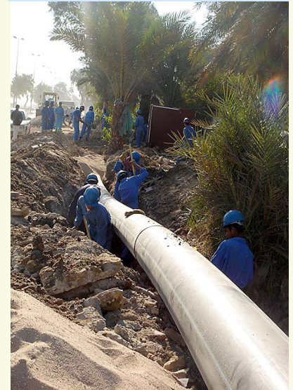
Iraqi civilians have installed 200 kilometers of water pipes made of high-density polyethylene.
