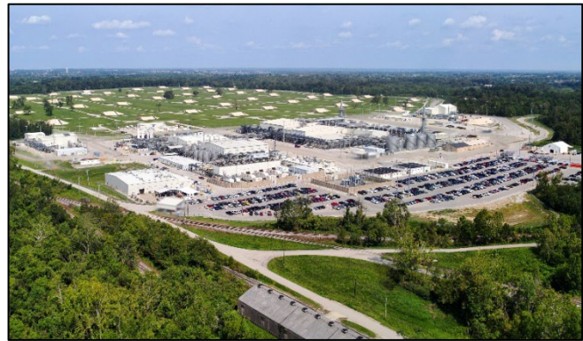
BGCAPP Facility Aerial Perspective
