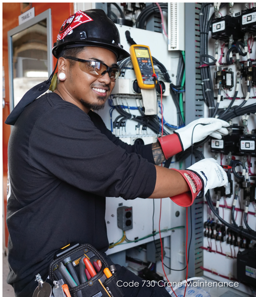
Code 730 Crane Maintenance Electrical Apprentice Joshua Chinen performs an initial voltage verification on a portal crane circuit board.
