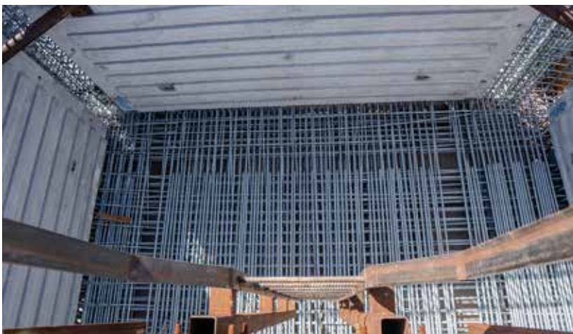
View from the top of a floor unit looking down at the rebar comprising the bottom of a typical cell prior to the concrete pour. Each unit is divided into 24 sections.
