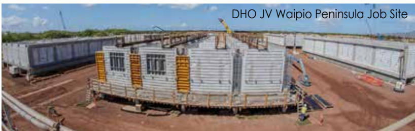
View from the top of a floor unit looking at other floor units in various stages of construction. The project includes nine 75'x127'x17' floor units that will make up the floor of Dry Dock 5.
