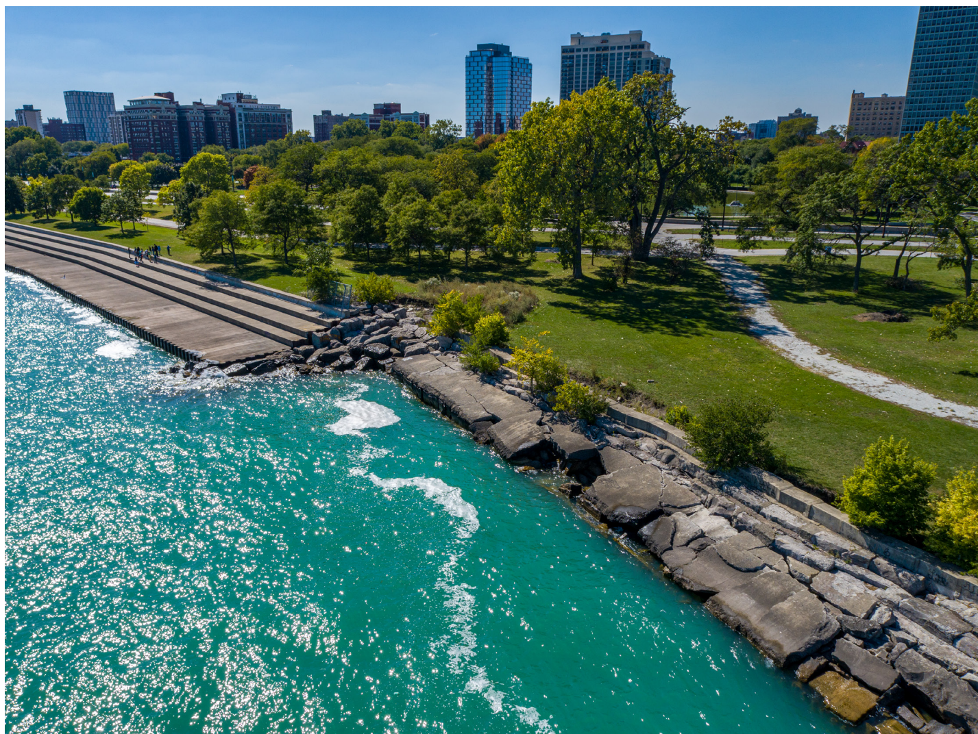
Lakefront edge at 51st St terminates without connection to trail
