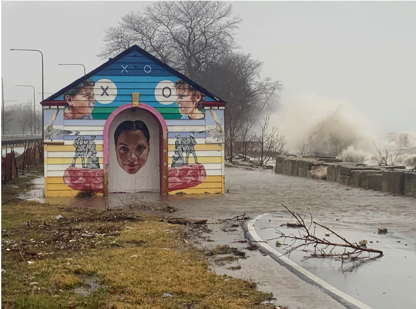
Existing restroom building located below FEMA flood elevation
