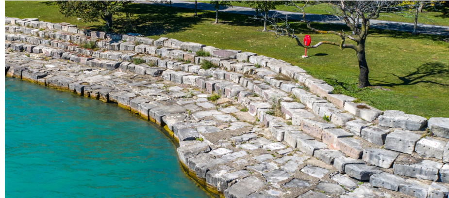
Stepped Stone Revetment
