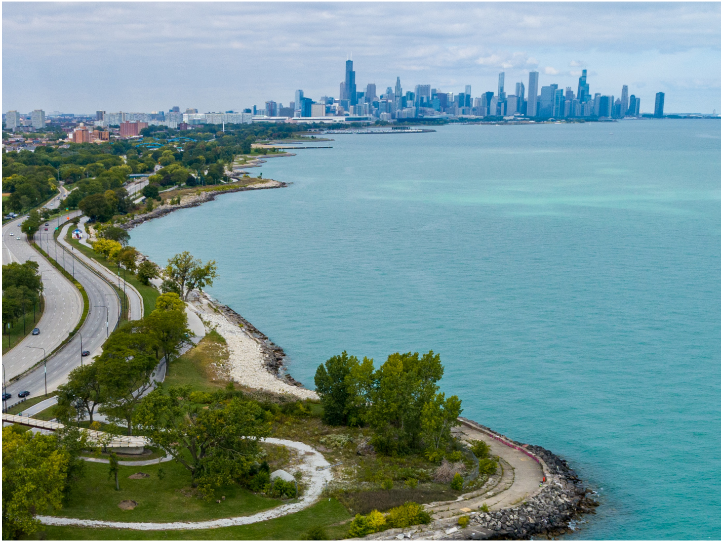
Aerial of Morgan Shoal project area
