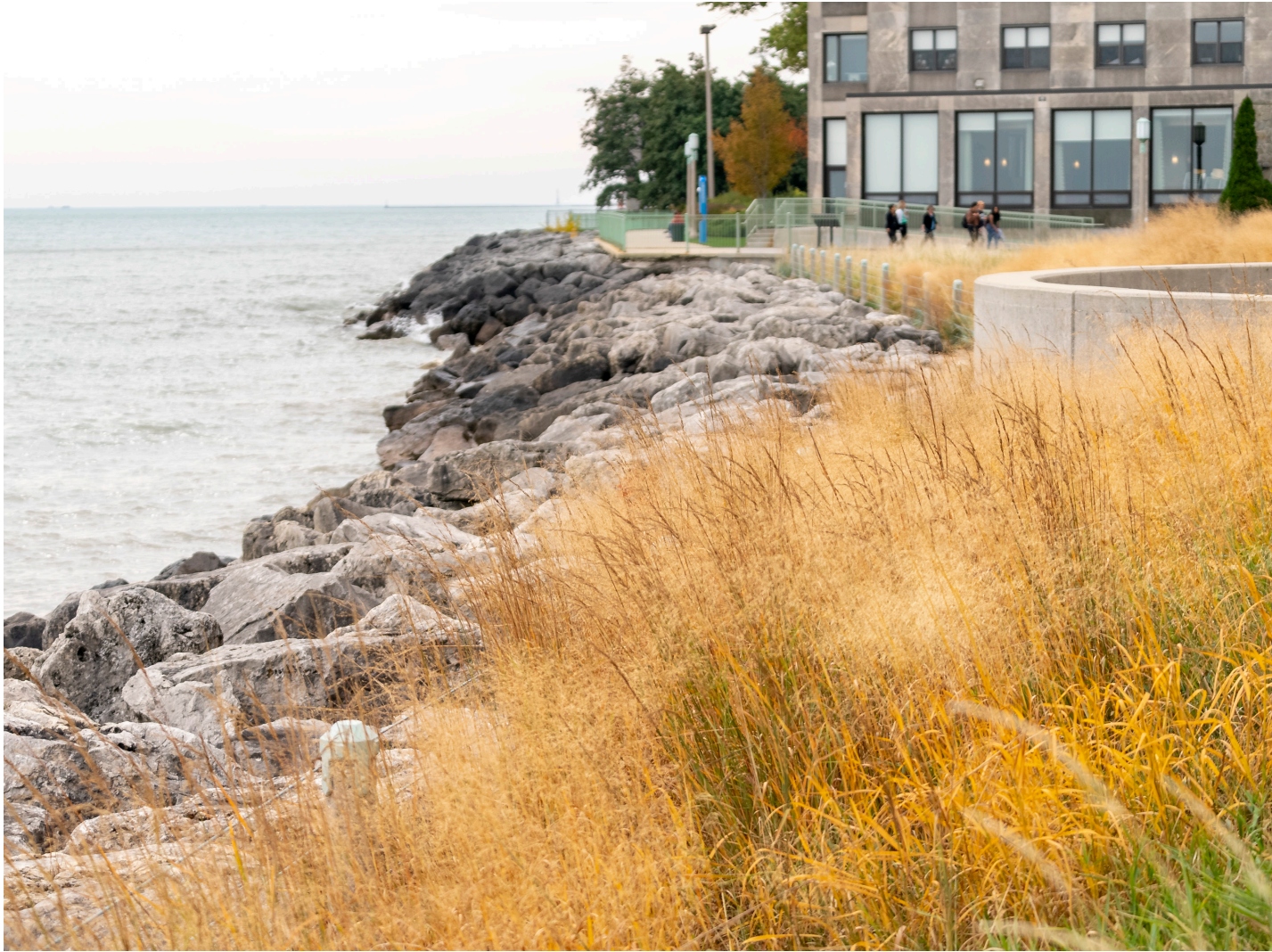
Loyola University Armor Stone Sloped Stone Revetment
