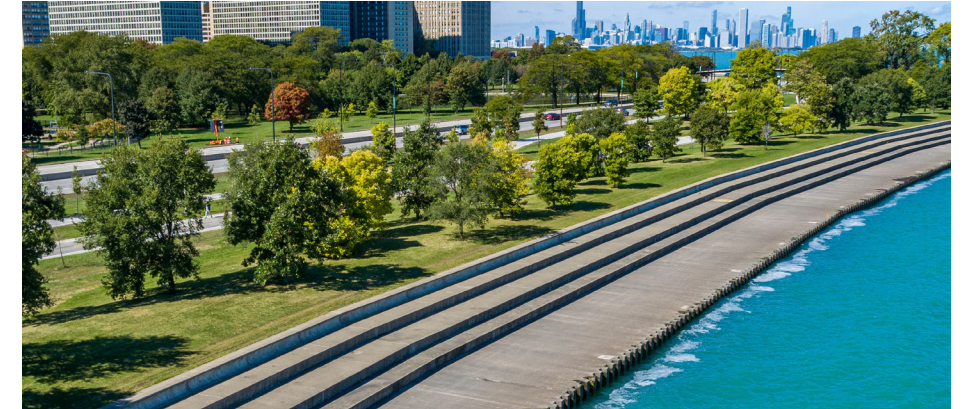
Stepped Concrete Revetment
