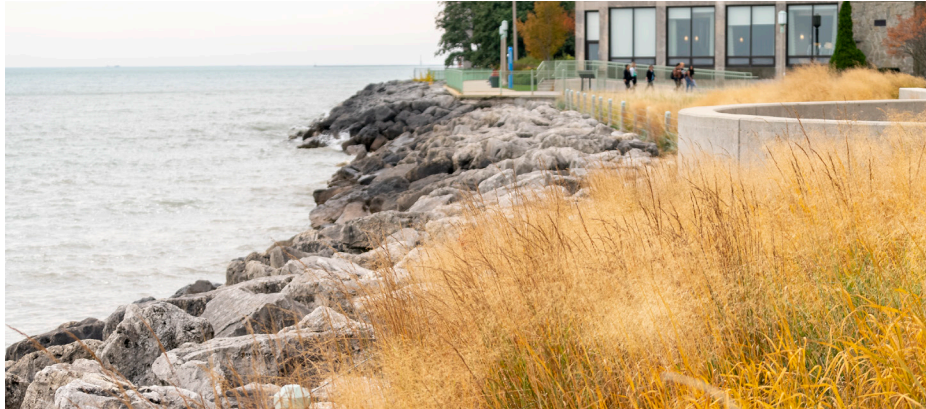
Sloped Stone Revetment
