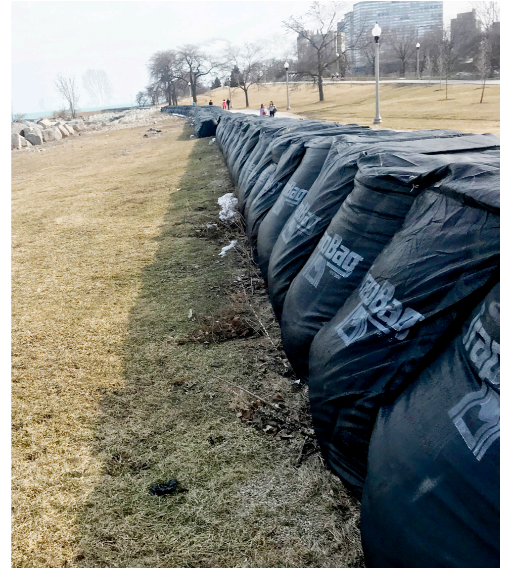
TrapBags installed as temporary flood protection
