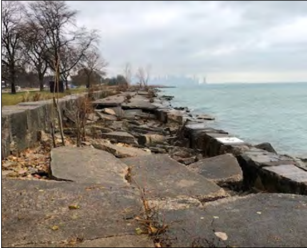
Figure 3: View of Existing Deteriorated Erosion Protection.
