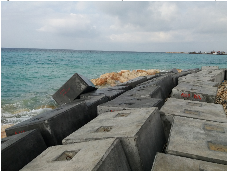
Figure 2: Unit Block Construction Subjected to Wave Forces and Uplift
