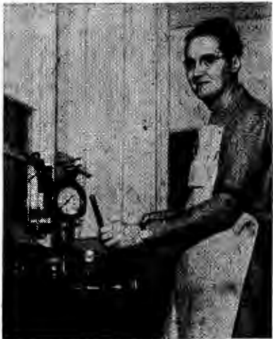
Testing an hydraulic pressure gauge, used with recoil mechanism in the field, is Leslie Evans.
