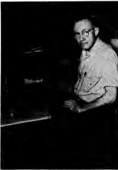
L. E. Hawkinson engraves a graduated scale for replacement in the mechanical instrument section.
