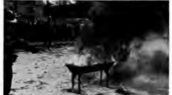
Mechanical foam is used on this oil fire, one of the many types of fires extinguished during week.
