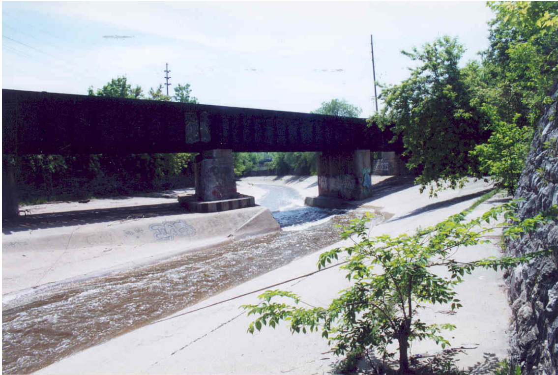
Figure 3 – Concrete lined Menomonee River Section
