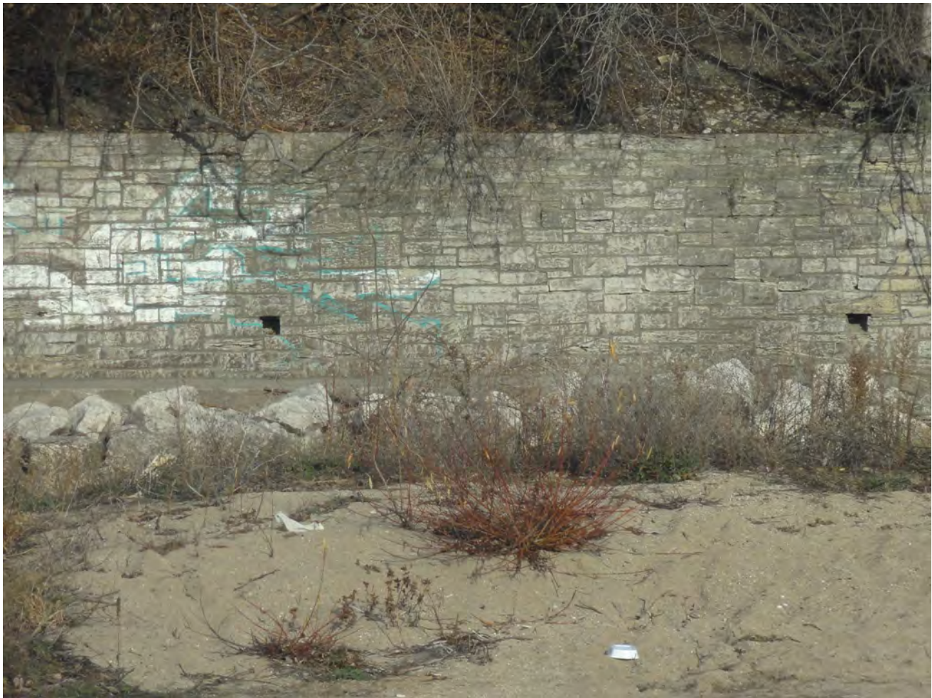
Figure 4. Existing WPA Wall in Background with Storm Drain Outfalls
