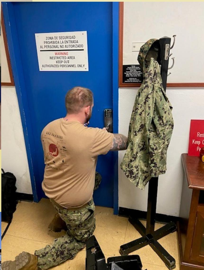
CM3(SCW/EXW) Christopher King is seen above removing an electronic cipher lock that stopped working. Efforts quickly enabled the five Marines to exit from a locked room.
