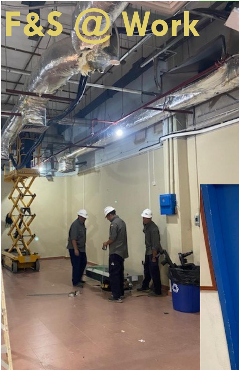
On the left you can see Facilities & Sustainment Team working on a project in BLDG 5, consisting of replacement of current HVAC system to accommodate an interior renovation for new residents of the facility. Numerous craftsmen from the F&S Branch met to discuss the timing of the phased tasks to be completed to ensure smooth operation on this renovation.
