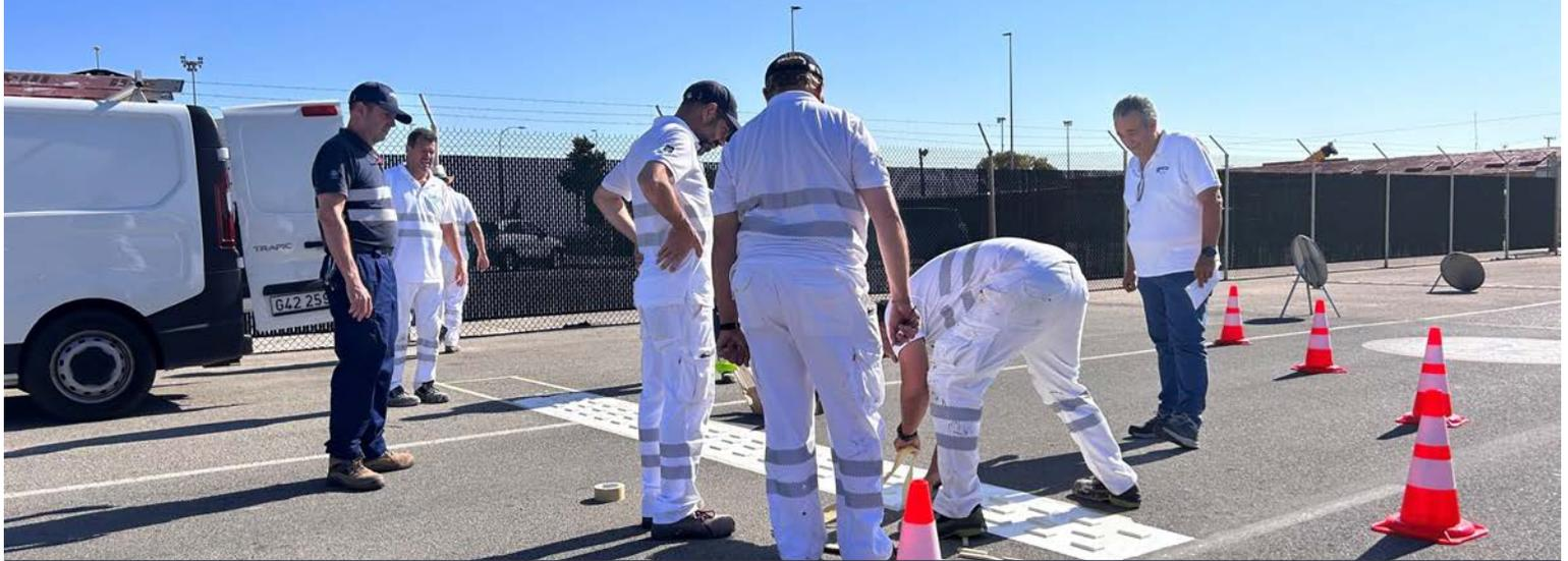
PWD Rota's Facilities & Sustainment Branch personnel are seen here installing a trial speed bumps in front of 158 of PWD Rota complex, under supervision by Rafael Lopez Puyana on July 25th, 2023. After the test bumps pass the tests, more of these are expected to be installed throughout the base, especially around the roundabouts, in order to alert the drivers and mitigate traffic accidents. - Photo and Article by LT Chanhon Lee
