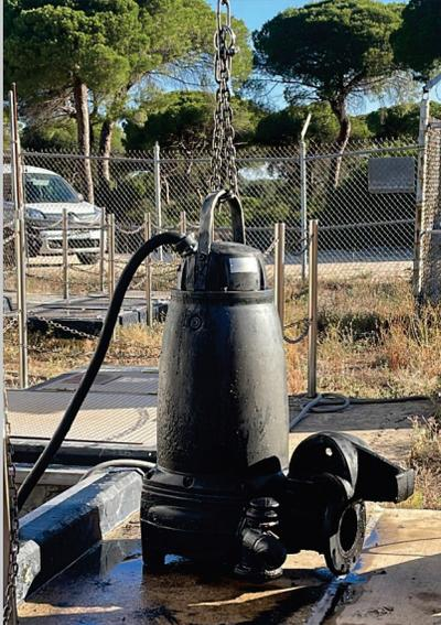
Not everybody has the guts to deal with dirty jobs, but someone has to do it. On 13 July, UEM and Crane Crew teamed up to remove the lift pump from Lift Station #9. Lift Pumps are used to ensure that wastewater is able to safely be transported from your drain to the treatment plant.
