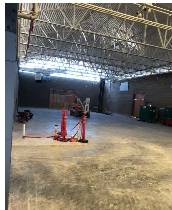
Working with Naval Support Complex Smokey Point officials, DCMA Seattle's relocation team transitioned personnel from its downtown Bellevue, Wash., office to the newly renovated space Aug. 10, 2020.
