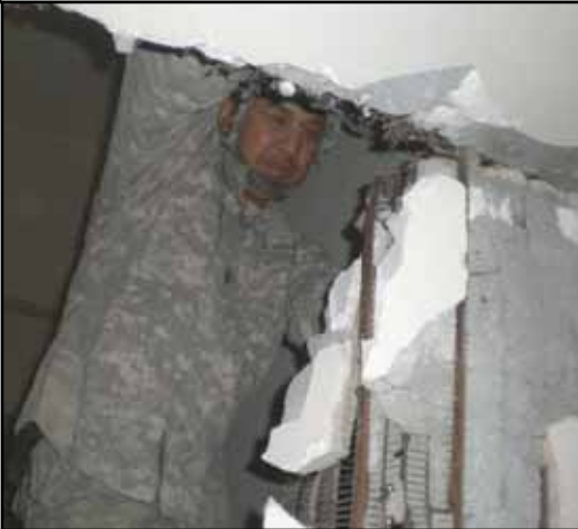
SGT Nakhonexay demolishes a bad ceiling of plaster, 4 April.
