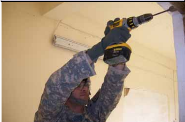
SPC Ammari drills a hole in a door frame so electrical cable can be run through.
