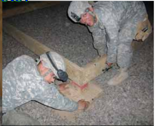
SPC Kleinheider & SPC Myers place footers for a Dining Facility.
