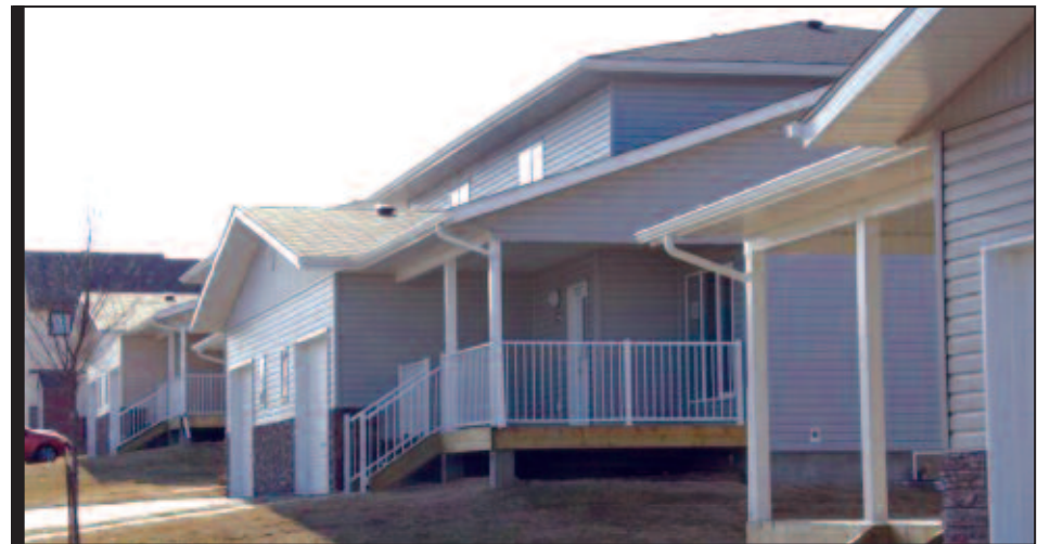
New PMQs await occupants at CFB Wainwright.
