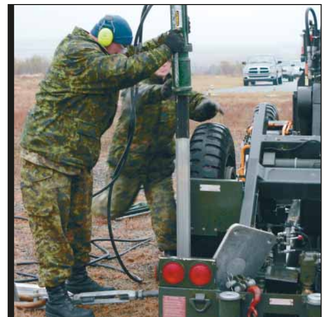
Students use the hydraulic stake driver to drive aluminum anchor stakes for the MAAS.
