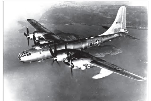
A Boeing B-50D Superfortress in flight wearing natural metal. The larger tail of the B-50 compared to the original B-29 can be seen here.
