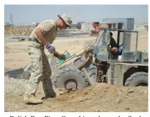
Polish Pvt. Piotr Oparski works on the final touches of a culvert as a scoop loader hauls the rest of the dirt.
