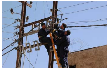
Iraqi workers trouble-shooting power lines. The CD program provides training for these types of repair activities. (GRD Photo)
