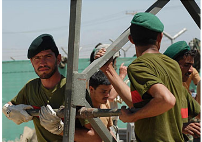
BUILDING A BRIDGE — Afghan National Army engineers of 4-3 Kandak, 201st Corps Command, assemble a 40-foot bridge section in preparation for emplacement of a Bailey Bridge during a future mission. (Photo by Capt. Ashley Dellavalle)
