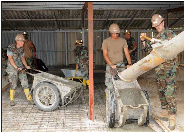
Det Senegal bees fill Georgia Buggies with fresh concrete on NAVSTA Rota.
