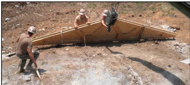
The ground crew prepares a gable end to be lifted by crane.
