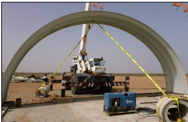
A crane crew assists the project crew with lifting the K-span into place.
