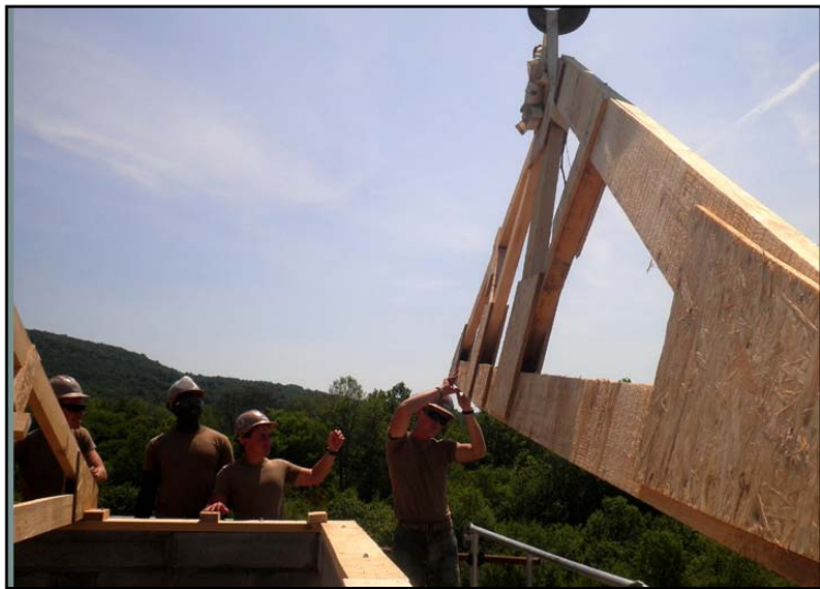
CM3 McKinney guides a truss onto the roof.
