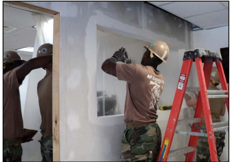
BU2 Pataky, BU3 Newell, BU3 Moore and CE3 Foster sanding and mudding the drywall at CTF-68 operations office.
