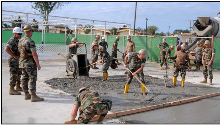
Det. Senegal bees pour concrete at a pool project on NAVSTA Rota.
