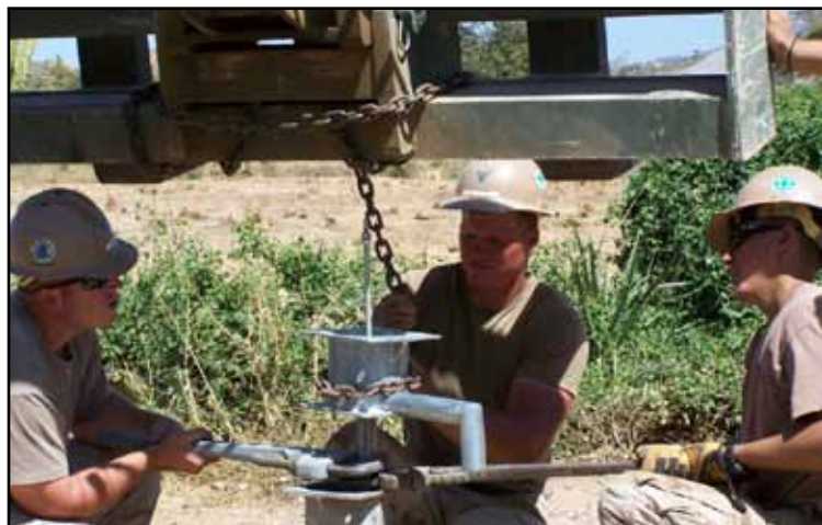
EO1 Hill, EO2 Helstrom and CM3 Durcholz lower the tank portion of the hand pump onto the draw pipe
