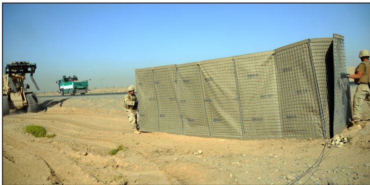
Two SeaBees with 21st Naval Mobile Construction Battalion out of Lakehurst, New Jersey, set up a Hesco Wall along Kandahar's Highway One as Combined Task Force Strike Soldiers from Company C, 1st Battalion, 502nd Infantry Regiment, provide security.
