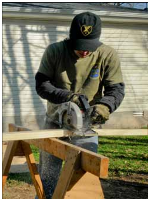
Sgt. Justin Higgason with Company B, 2nd Battalion, 502nd Infantry Regiment, cuts wood braces for use while installing walls at a Habitat For Humanity project in Hopkinsville, Ky., Dec. 10. Strike Force Soldiers assisted with the foundation installation and floor bracing.
