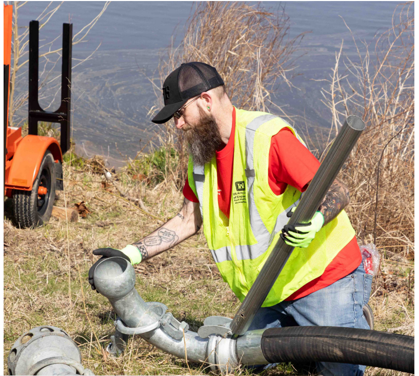
Top: Nick Bails demonstrates how to connect piping for a self powered water pump.
