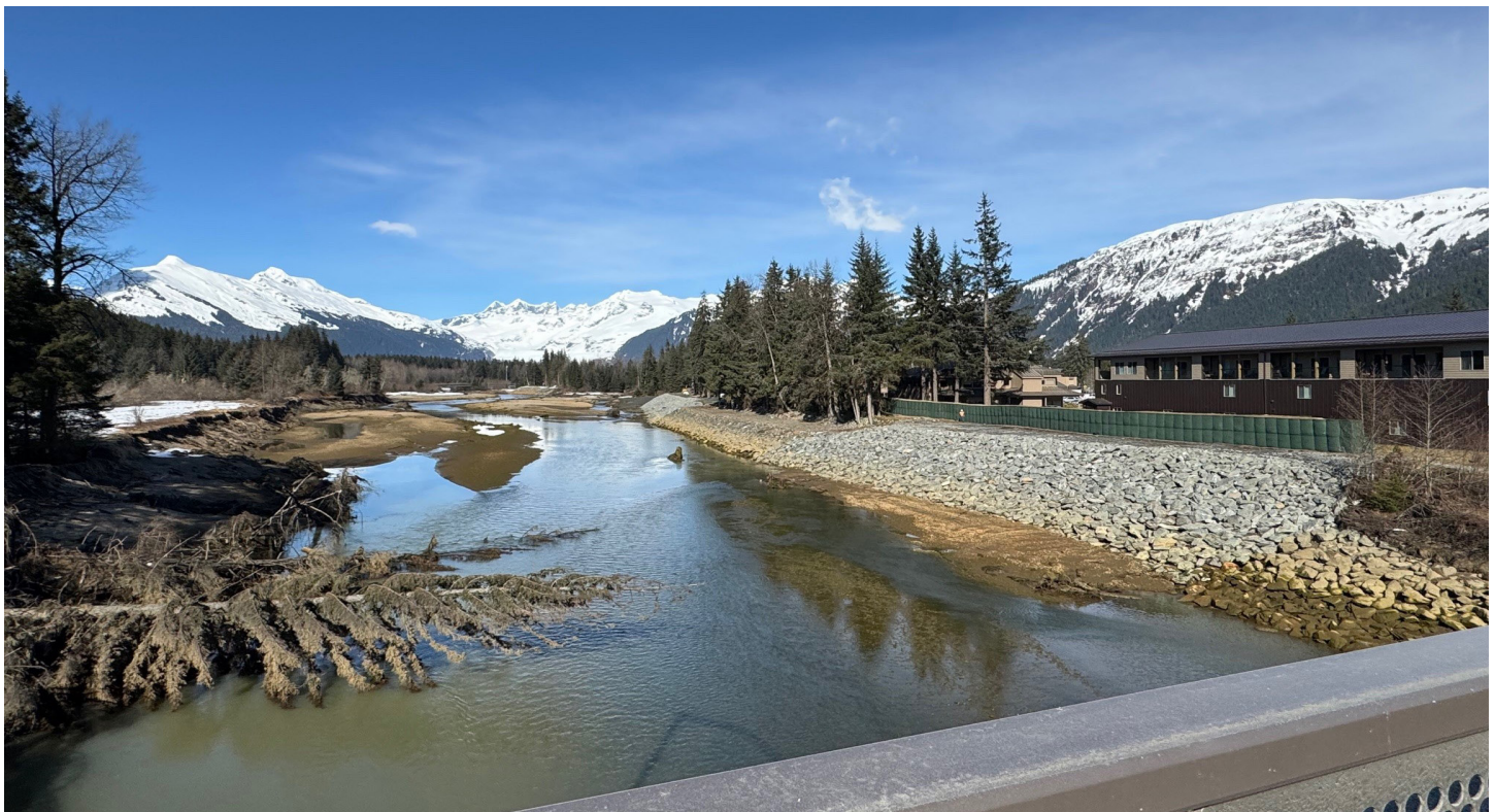
A Gabion basket wall protects homes and infrastructure along the Mendenhall River in Juneau, Alaska. This structure is critical for preventing erosion and diverting floodwaters caused by seasonal glacial outbursts. Courtesy Image
