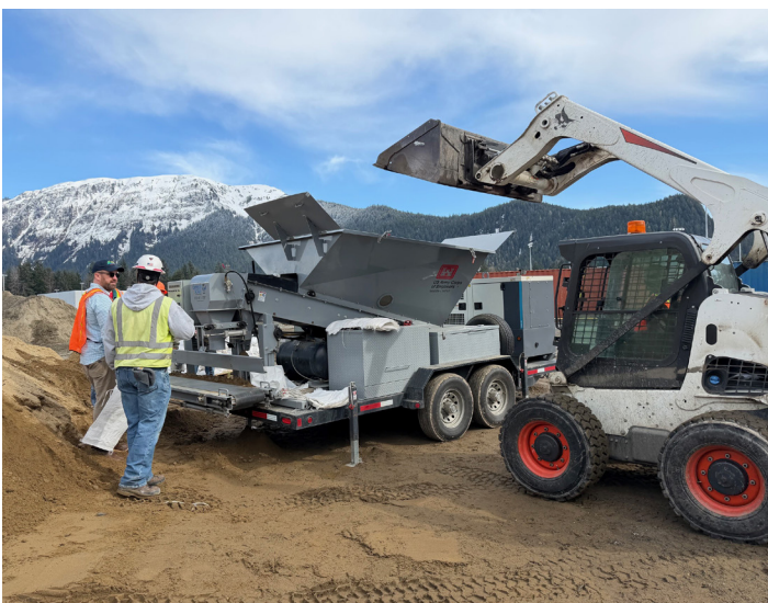
USACE volunteers, trained by Cory Haberman, instruct local volunteers on proper sandbag-filling techniques to help shore up the Mendenhall River. Courtesy Image
