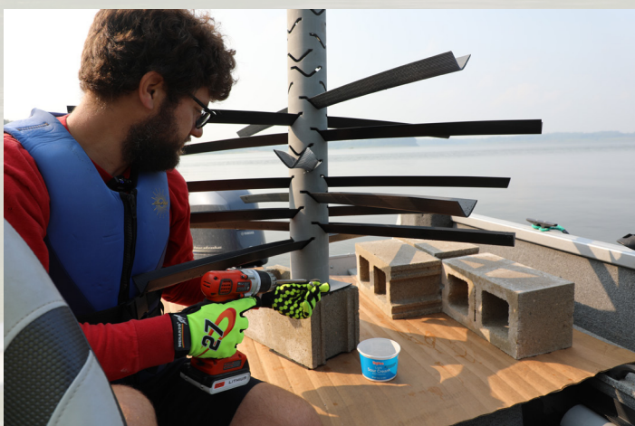
Josh Ellis, a Pella Middle School science teacher and summer extern with the U.S. Army Corps of Engineers, Rock Island District, at Lake Red Rock assembles a ‘safe haven’ artificial fish structure in the lake.
