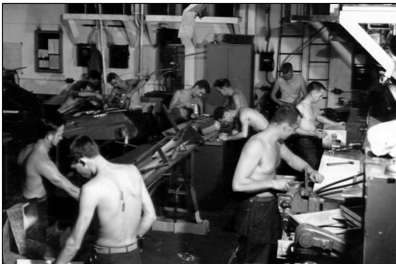
Figure 30: Sheet Metal shop manufactured and repaired all structural parts for aircraft.
