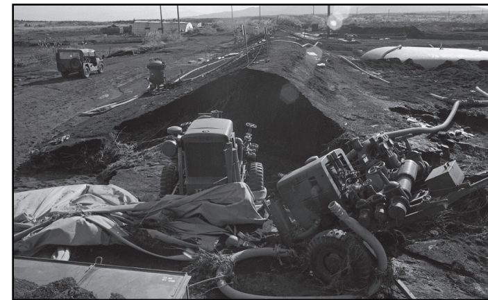
Photo of the breached berm. Courtesy of Stars and Stripes.
