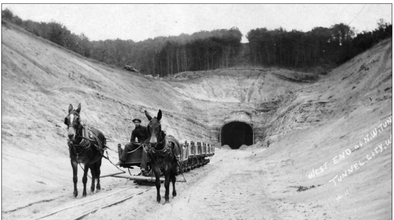
Photo shows construction work on the Chicago & North Western Railroad in Tunnel City, Wis., in 1911. Did you know that Monroe County has six railroad tunnels? Three are in Tunnel City and three are on what is now the Elroy-Sparta Bike Trail. This tunnel is located just a few miles from Fort McCoy.
