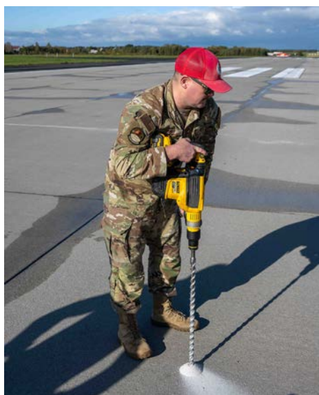
Master Sgt. Jordan Deady, 200th Rapid Engineer Deployable Heavy Operational Repair Squadron Engineer, drills a hole on a runway in preparation for a penetration test at Gdynia, Poland, Oct. 15.
