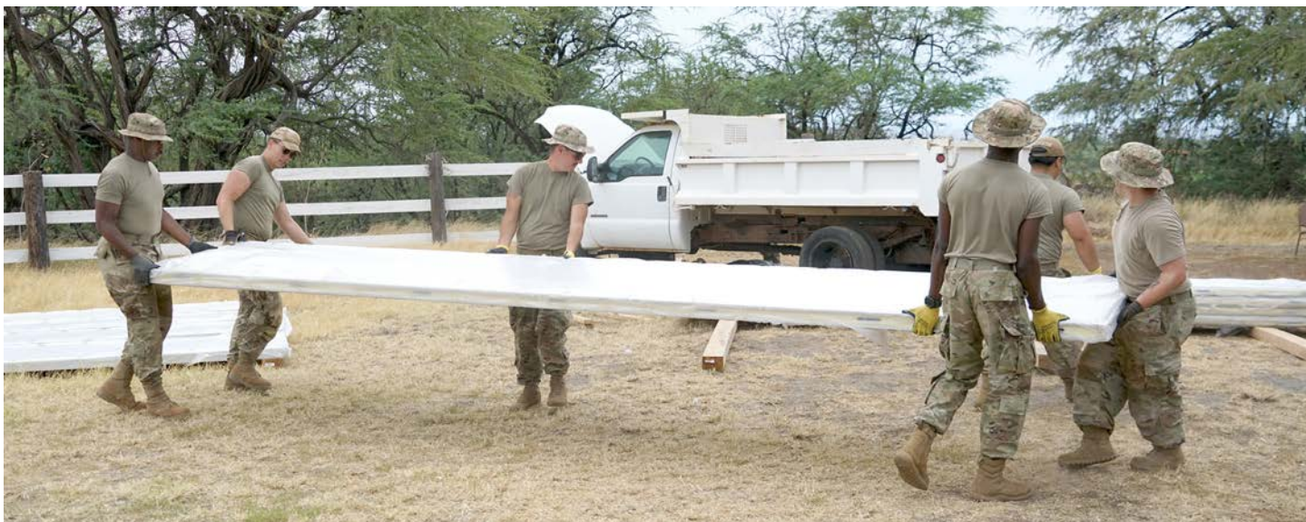
The 182nd Civil Engineer Squadron, Illinois Air National Guard wrapped up their Innovative Readiness Training (IRT) rotation at Pu‘uhonua ‘O Wai‘anae (The Village) in Wai‘anae, Hawai‘i in late June.
