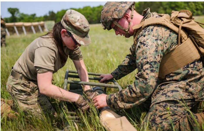
U.S. Air Force Airman 1st Class Toni Bussell, fuels specialist, 182nd Airlift Wing, Illinois Air National Guard, helps install a hose connection. The fitting connects all the hoses together as part of a tactical airfield fuel disposing system for the forward arming refueling point in support Sentry North 25, June 2.
