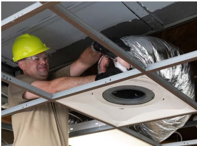
Tech. Sgt. Jeremy Reith, noncommissioned officer in charge of heating, ventilation and air conditioning, 126th Civil Engineering Squadron, secures a flexible duct air supply to a drop ceiling air diffuser on Aug. 2, at the Atlantic City Air National Guard Base in Egg Harbor Township, New Jersey.
