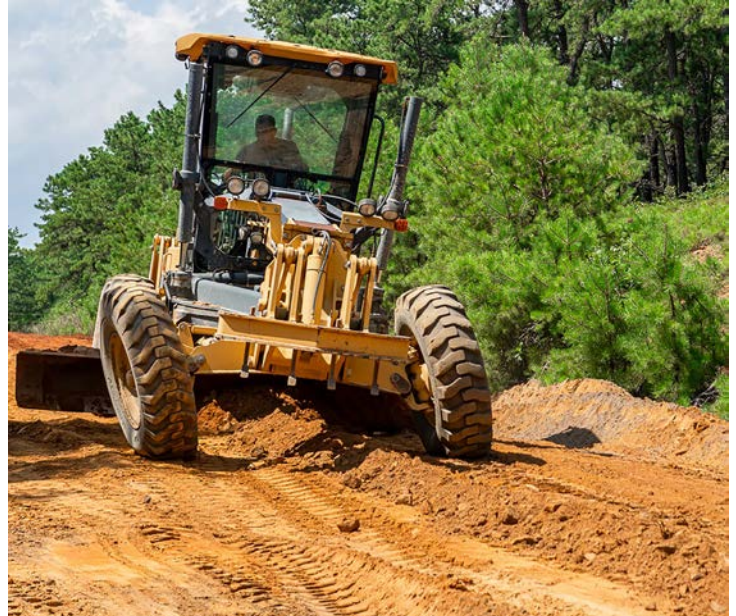
Senior Airman Todd Schulte, pavements and construction equipment operator of the 126th Civil Engineering Squadron, operates a 670D Grader on Aug. 2, as he applies the final grade on an unimproved road to ensure proper water drainage.
