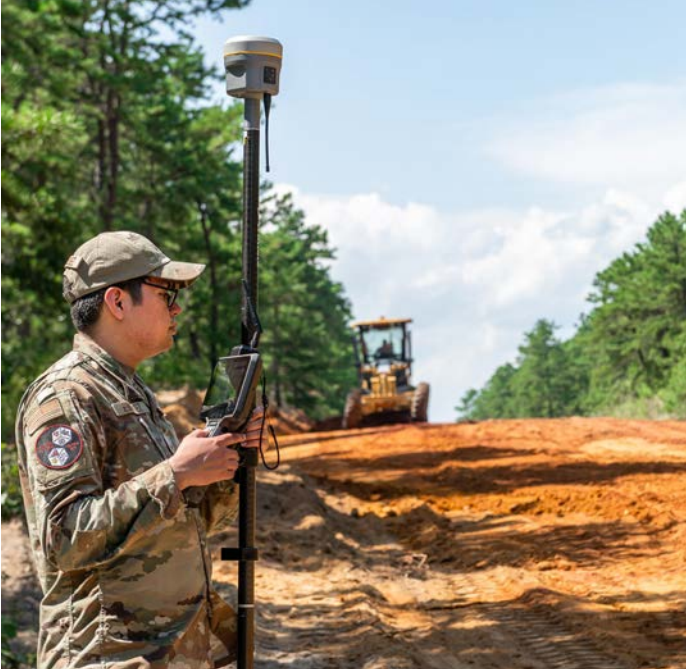
Airman 1st Class Johnathan Enriquez, engineering journeyman, 126th Civil Engineering Squadron, operates a Trimble R12i Global Navigation Satellite System rover at Warren Grove, New Jersey, Aug. 2. Enriquez performed a topographic survey to capture the grade of the repaired road.
