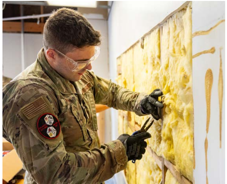
Senior Airman Jacob Maas, electrical, 126th Civil Engineering Squadron, installs wiring that will provide power to receptacles in the 177th Fighter Wing's egress shop Aug. 3, at Atlantic City Air National Guard Base in Egg Harbor Township, New Jersey.
