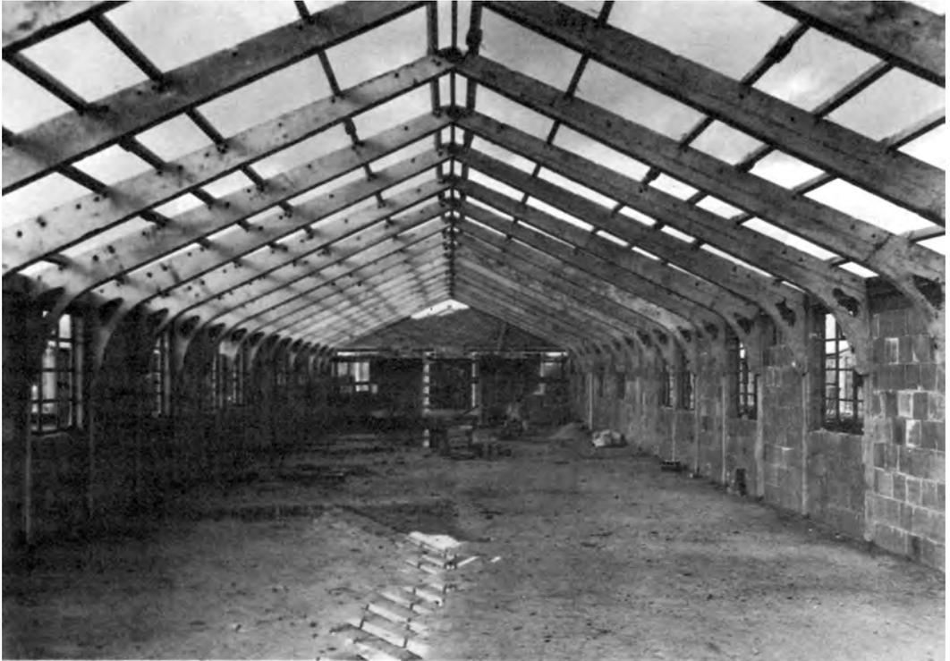
HOSPITAL CONSTRUCTION EMPLOYING PREFABRICATED CONCRETE ROOF TRUSSES
