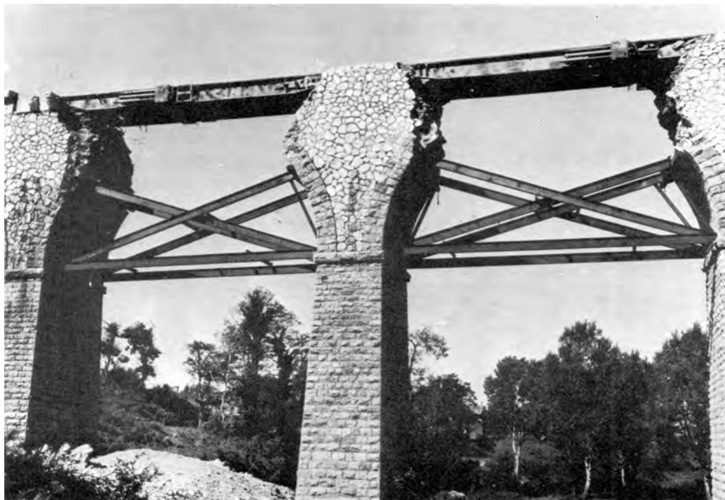
THE AIX BRIDGE, WHICH USED THE CARRIAGE OF A GERMAN RAILWAY GUN
