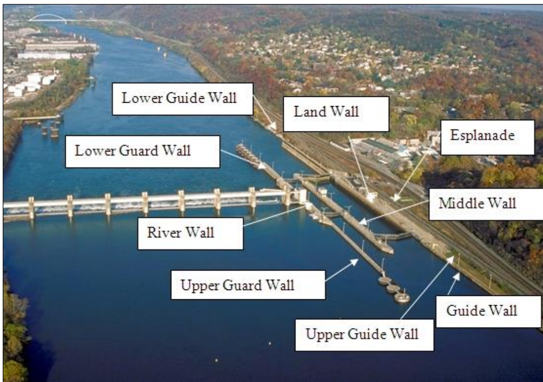
Photo 4-1: Lock Wall Component Nomenclature
