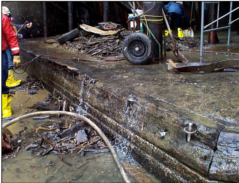
Photo 4-2: Miter Gate Sill, Emsworth Auxiliary Chamber
