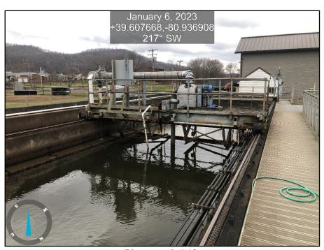
**Photograph # 12** WWTP, clarifier machinery
