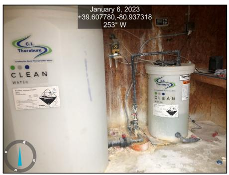
Photograph # 21 WWTP, sodium bisulfate tank
