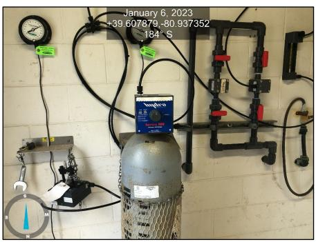
**Photograph # 19** WWTP, chlorine diffuser
