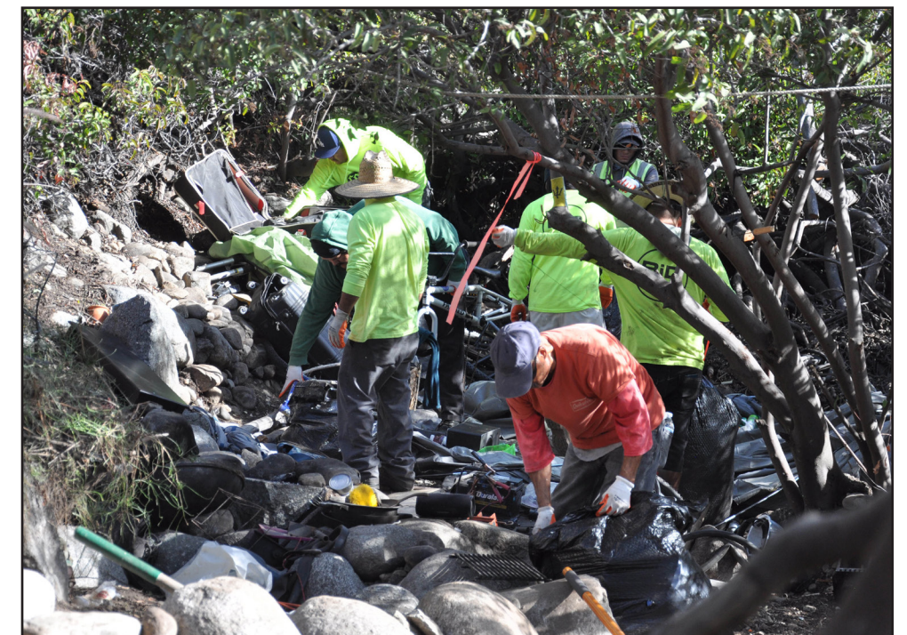
Workers contracted by the U.S. Army Corps of Engineers Los Angeles District remove trash and debris from the riverbed of the San Gabriel River Dec. 4 near Azusa, California. The cleanup took place over a three-week period after bird-nesting season ended.
