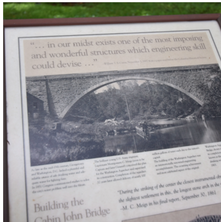
The Cabin John Bridge was the longest single-span masonry arch in the world from 1864-1903. (U.S. Army photos by Cynthia Mitchell)
