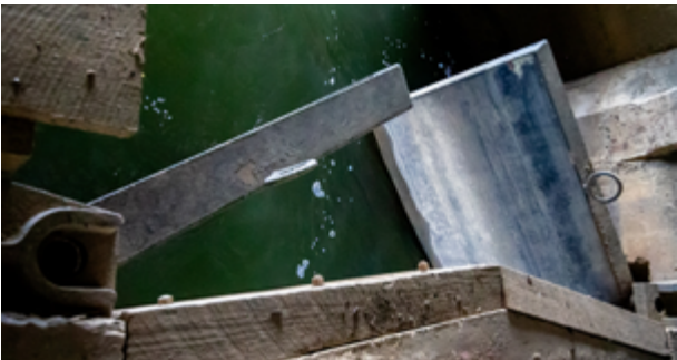
(Above) A view of the Washington Monument from below the Tidal Basin Inlet Bridge. (Right) The gates are designed to operate with the rise and fall of the tides. The inlet gates open to allow water from the Potomac River to enter the Tidal Basin during the rising tide. When the tide is falling the water pushes these gates closed and the outlet gates open on the Washington Channel. (U.S. Army photos by Christopher Fincham)
