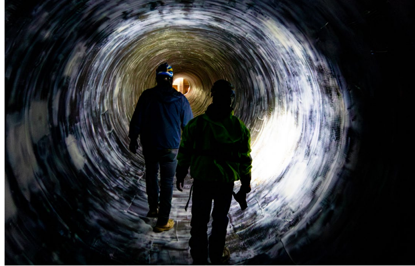
Teammates walk inside the Old Conduit inspecting newly installed carbon fiber. (U.S. Army photos by Christopher Fincham)
