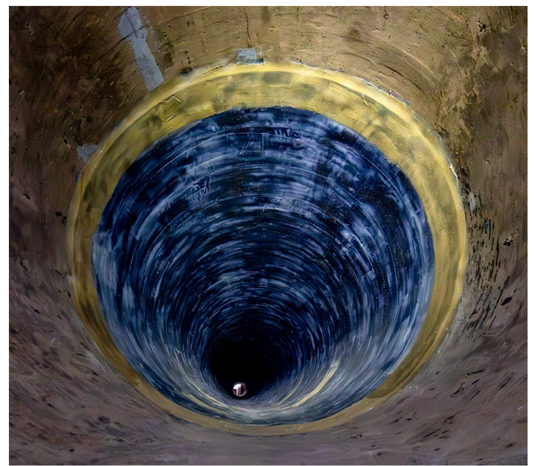
(Above) A teammate points out where the newly installed carbon fiber meets the original material of the conduit.
